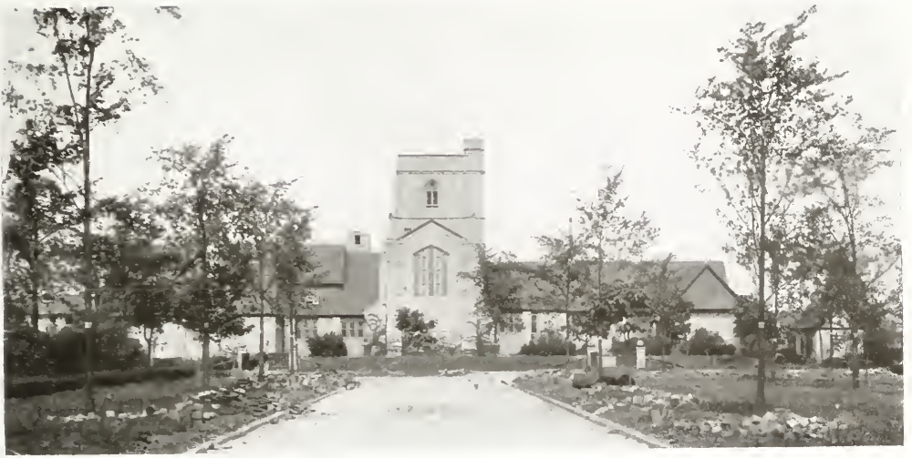
EXTERIOR—ST. MARY'S CHURCH.
